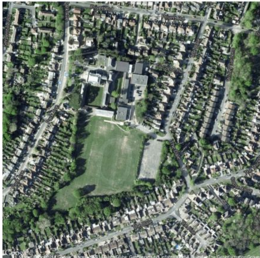
Aerial view of site and context
