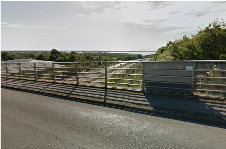
Bridge further east of site
