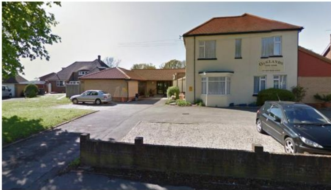
Fig. 5: View from Stakes Hill Road. (Google Streetview)
