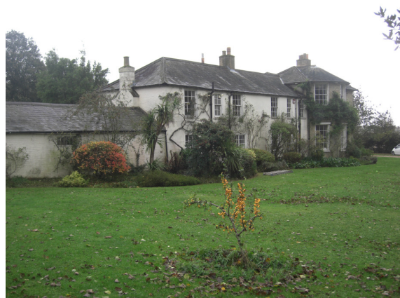
West elevation - approach from the drive
