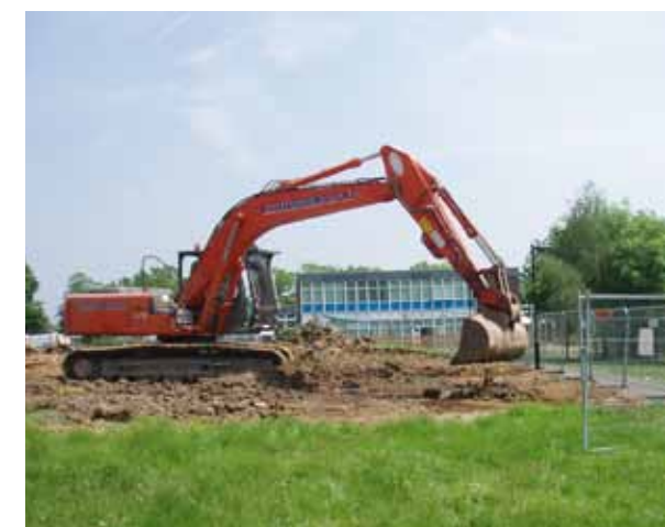
Figure 19: Demolition of Meadowlands Infant School 2009
