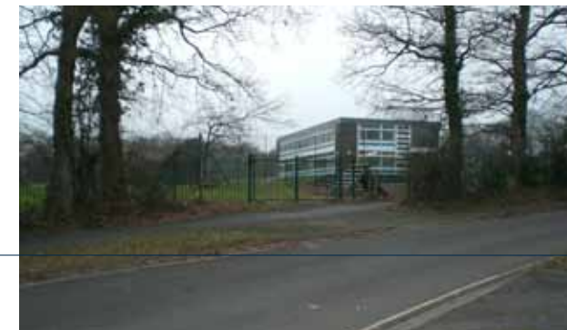
View 5: Gated access and dropped kerb on Woodcroft Lane
