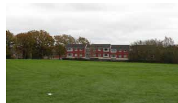
View 6: Looking east towards flats in Renown Gardens
