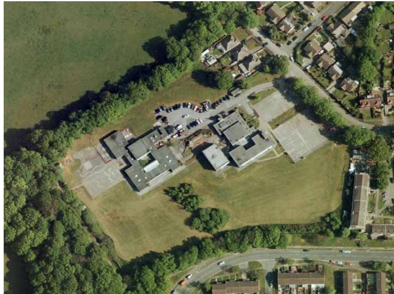
Figure 3: Original site of the former Meadowlands Infant and Primary Schools
