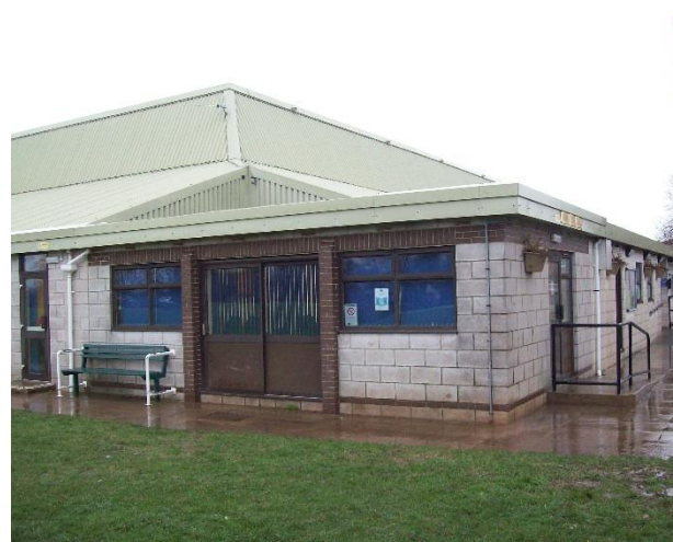
Figure 6- Existing South Façade
