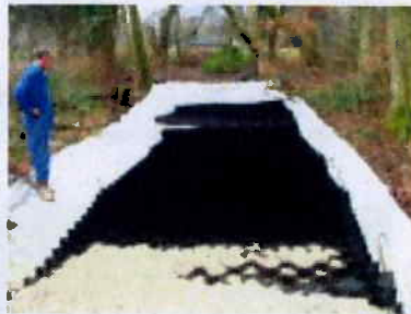
Installation of the CellWeb™ system.
