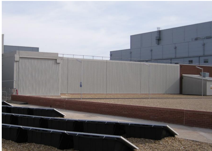
Fig.3 - Existing building with High Bay warehouse in the background.
