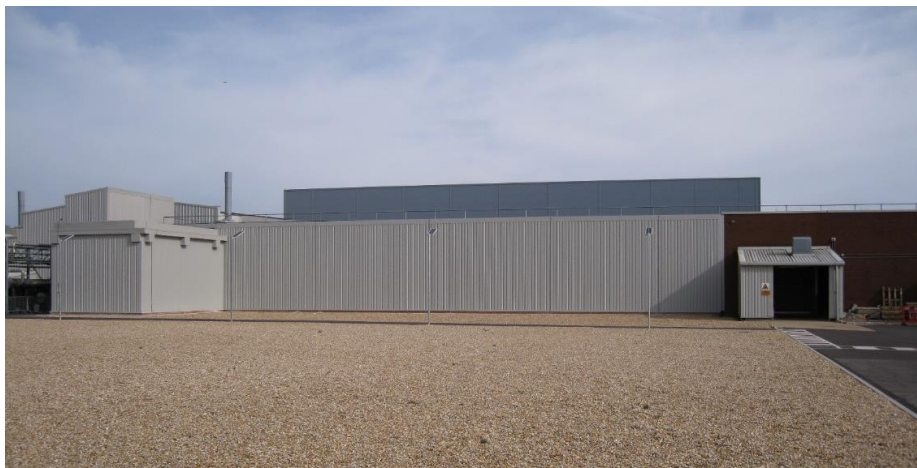
Fig. 2 - Existing Building (Front view – West Eleavtion)
