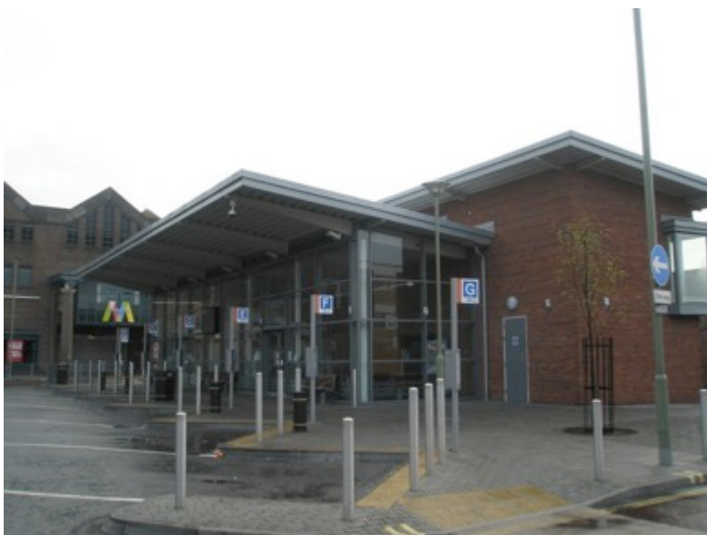
Existing Bus Terminal
