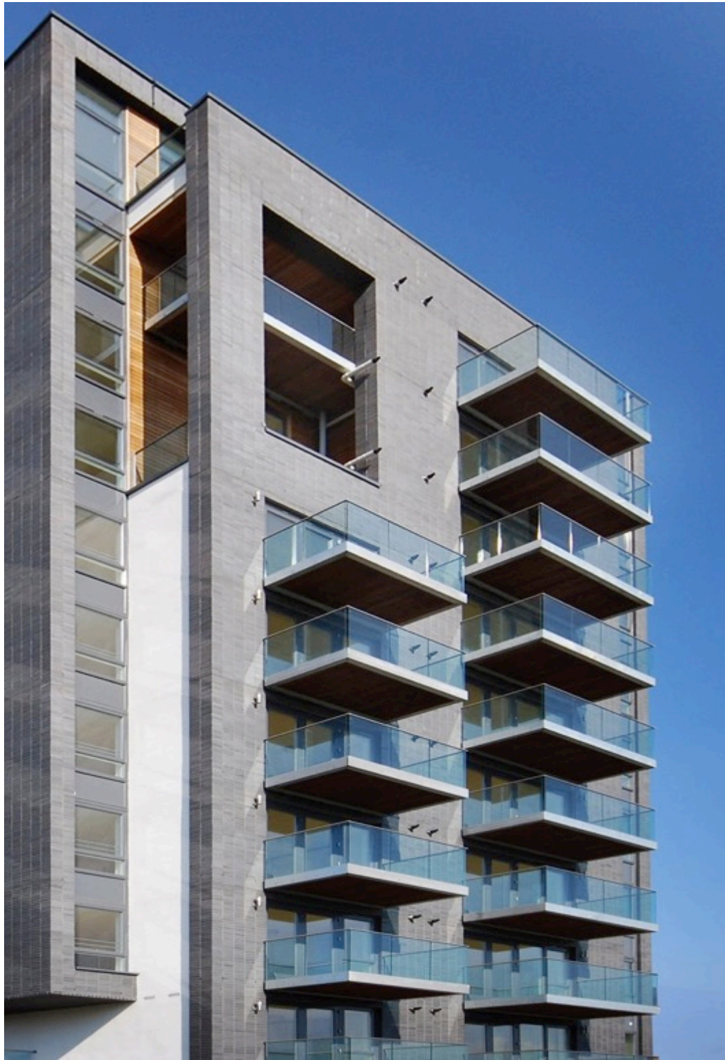
Facing Brick with amenity balconies and inset openings
