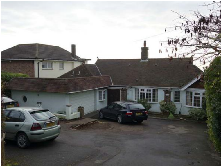
FRONT VIEW (NE)
