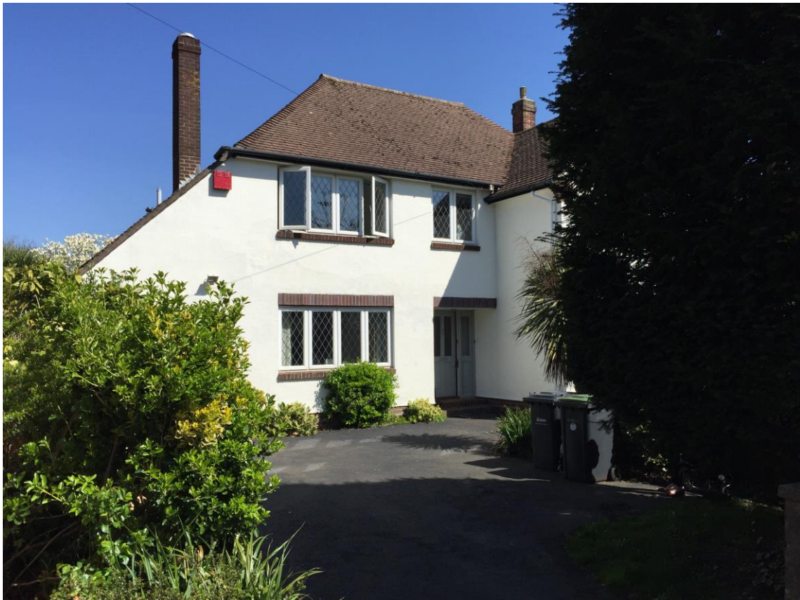
Figure 1: View of property
