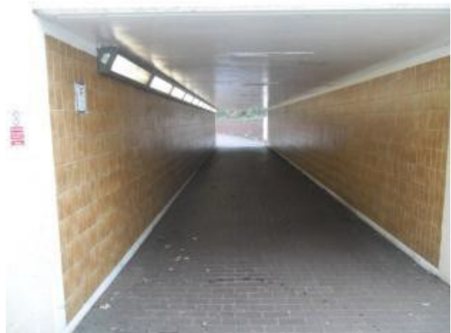
Photo 4.2: Maurepas Way underpass
