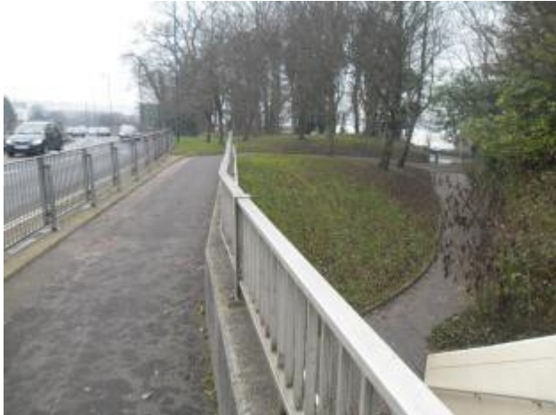
Photo 4.1: Access ramp to Maurepas Way underpass
