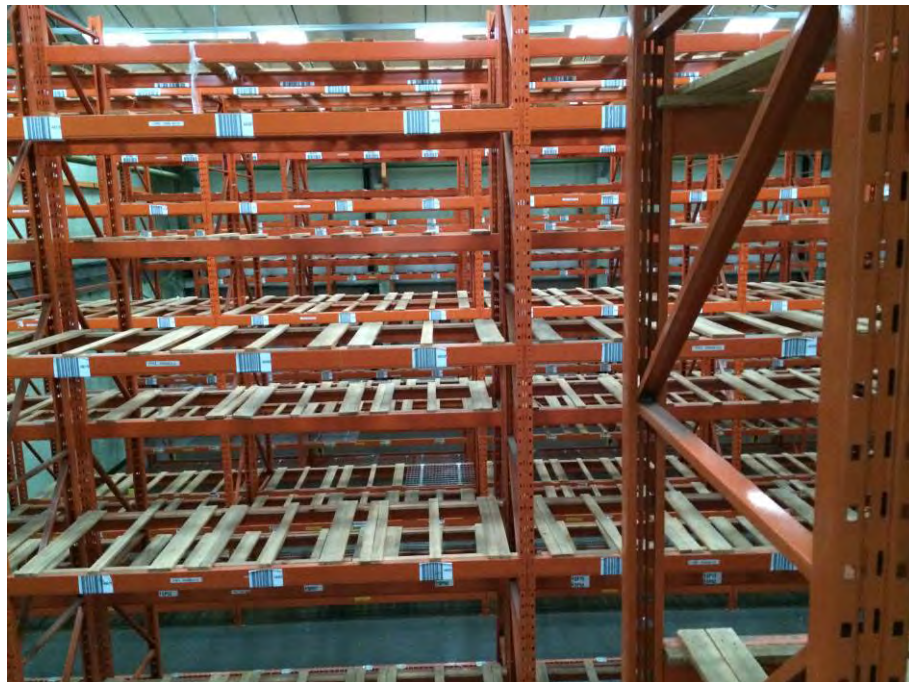
Photograph 6 – Racking area within the central section of Building 1
