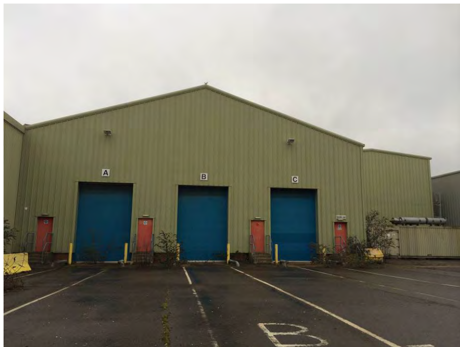
Photograph 14 – Factory doors on southern aspect of Building 1
