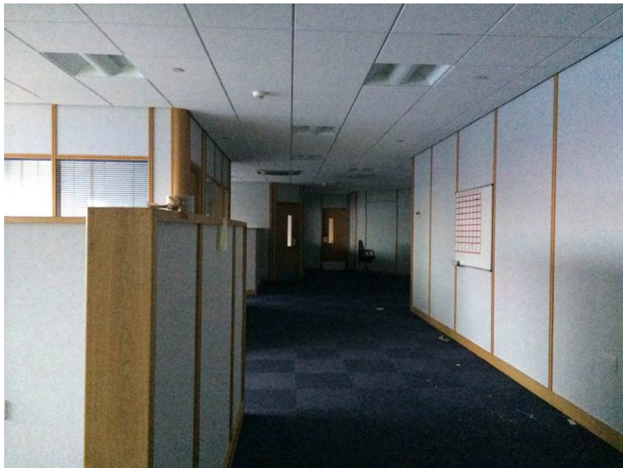
Photograph 8 – Offices within Building 1
