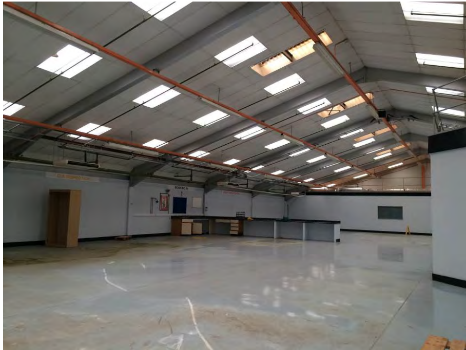
Photograph 7 – Warehousing area within Building 1
