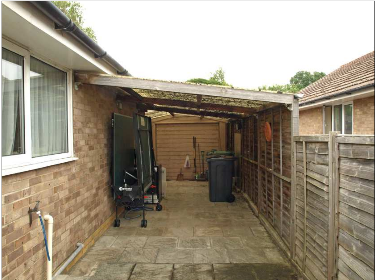
Front of existing garage and lean-to covered area
