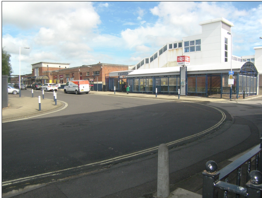
Plate 1: View of Havant railway station from the south-east
