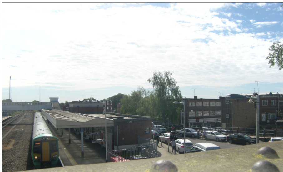
Plate 2: View from north-west taken on passenger footbridge at Havant railway station
