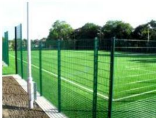
Example of ball-stop fencing
