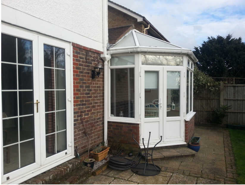
Existing conservatory to be removed and replaced with more solid structure.
