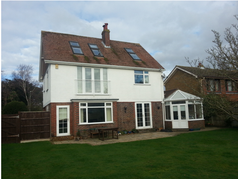
Existing Rear of building
