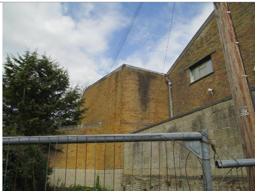
Plate 3: Rear of main workshop buildings
