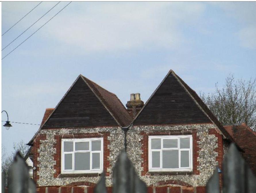
Plate 6: Main eastern elevation with timber panels
