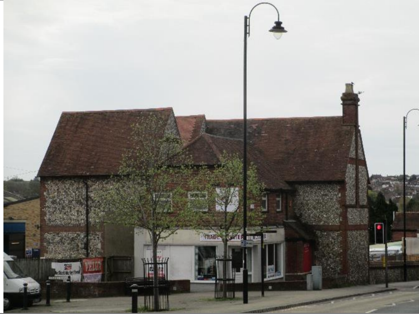
Plate 5: Main office building in north west corner
