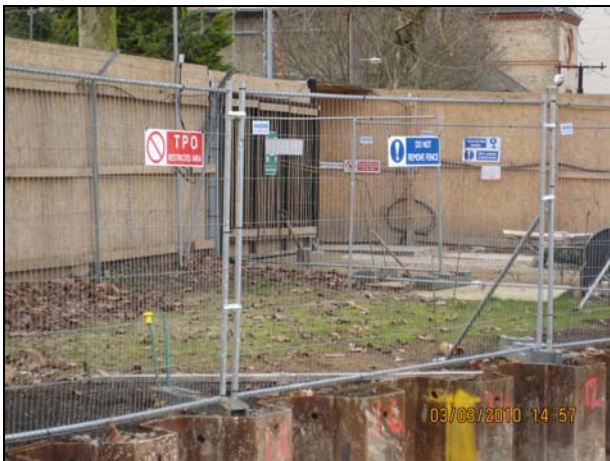
Fencing and signage around protected tree
