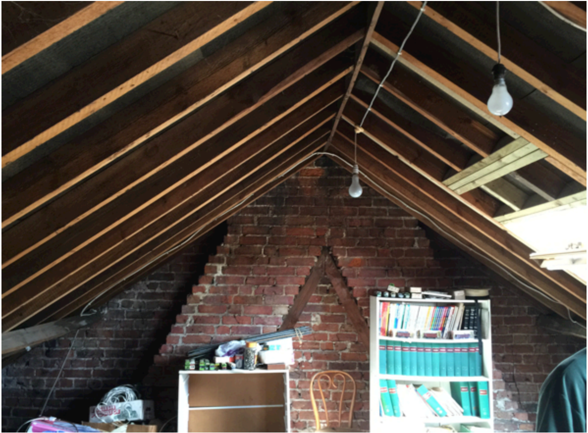
Figure 3. The well lit roof void of this property.
