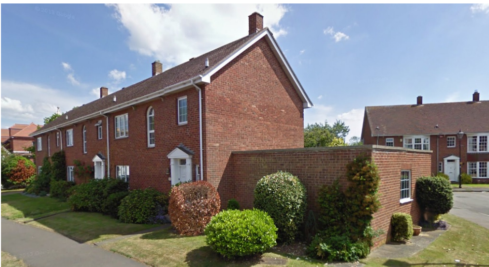
Corner opposite site
