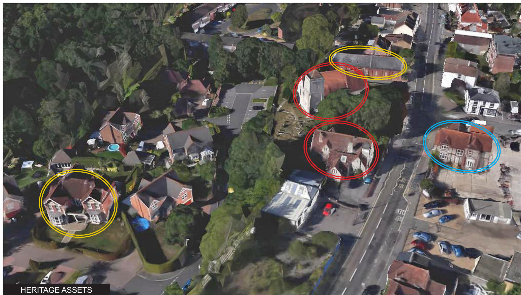
Oblique aerial photograph showing listed buildings circled in red; the non designated heritage assets in yellow and the former Vicarage on the application site in blue.
