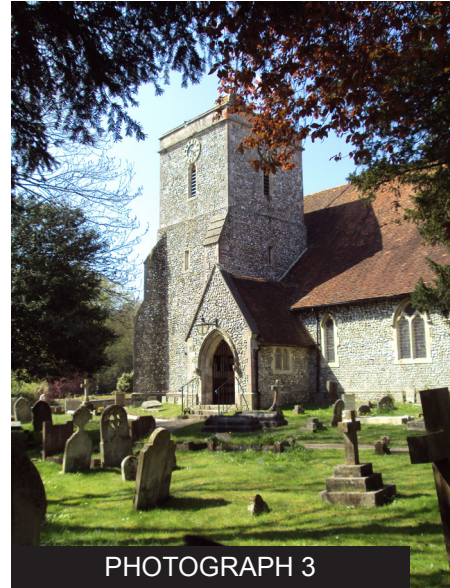
The south side of St John's Church (which is a grade II listed building) overlooking the graveyard.
