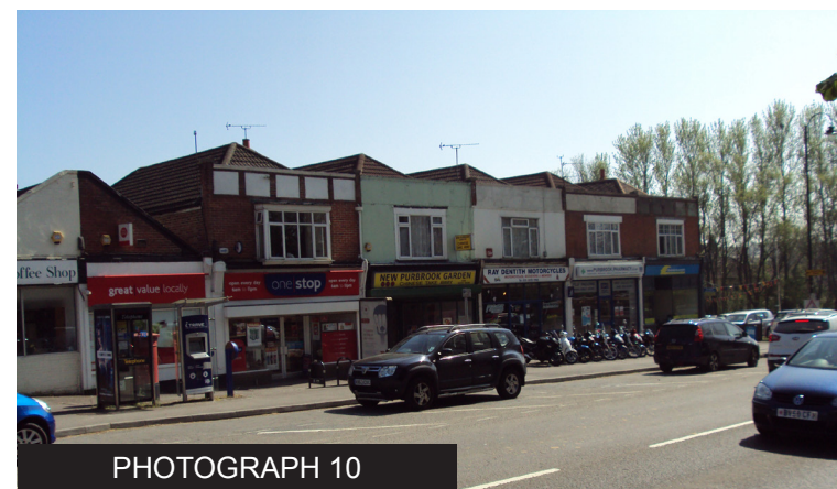
The east side of London Road to the south of the application site.
