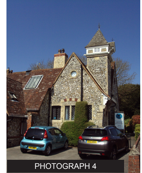
The south elevation of the former National School (again a grade II listed building) seen from London Road.
