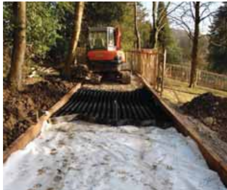
Fallbarrow Park, Windermere: CellWeb TRP® Installation
