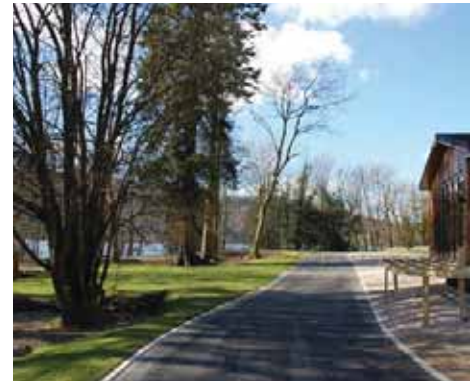
Fallbarrow Park, Windermere: Completed CellWeb TRP® Installation
