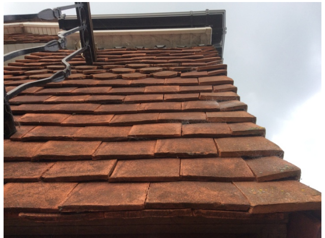
Figure 5. The hanging tiles devoid of evidence to suggest the use by crevice roosting bats roosting upon the eastern elevation of 40 Bath Road.
