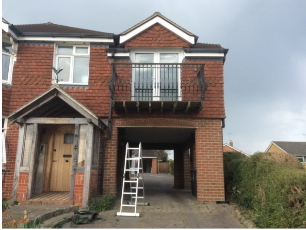
Figure 2. East facing aspect of 40 Bath Road, with the area proposed for alteration above the car port and to the right of the porch.
