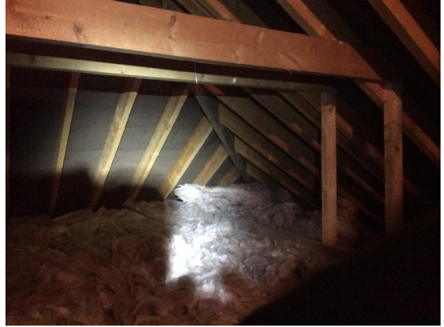
Figure 3. The roof void within 40 Bath Road, timber framed with bitumen roofing felt.
