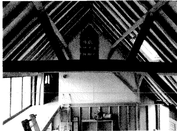
The first-floor bedroom in the northern part of Antrims Barn.
