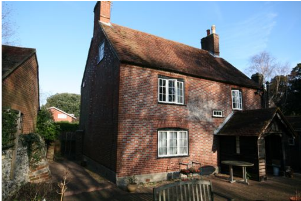
View looking north showing the site of the proposed extension
