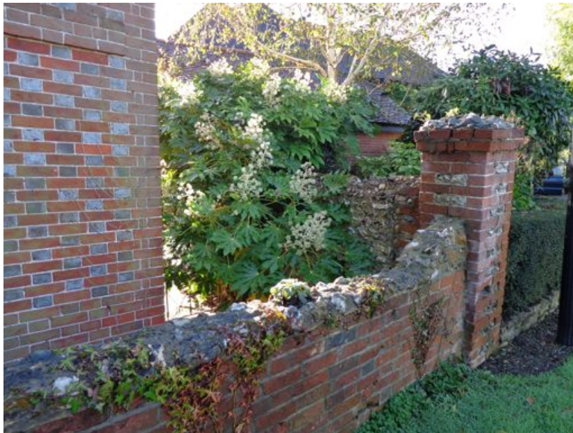
View of the boundary wall to the road, which will not be affected by the works.
