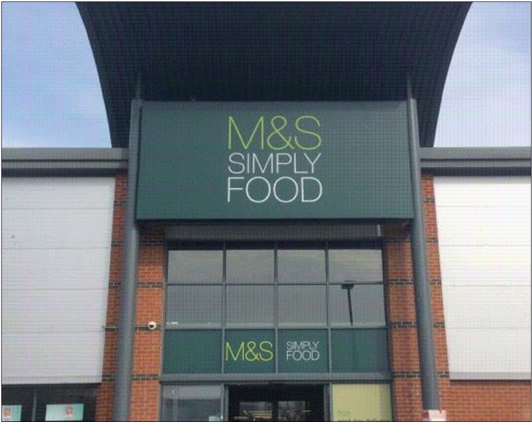
Entrance elevation existing signs
