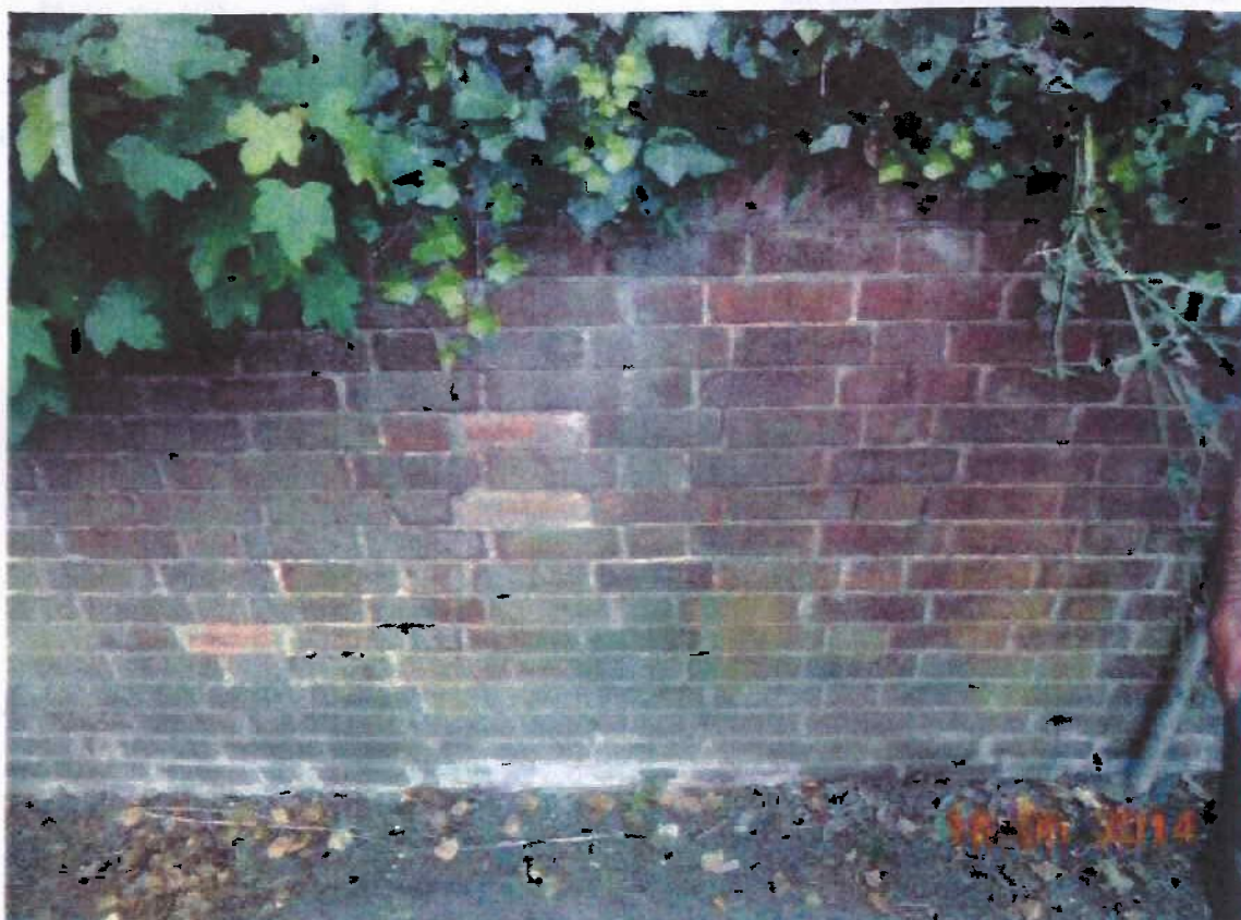
Photo No. 03 – Area where trial hole excavated behind wall
