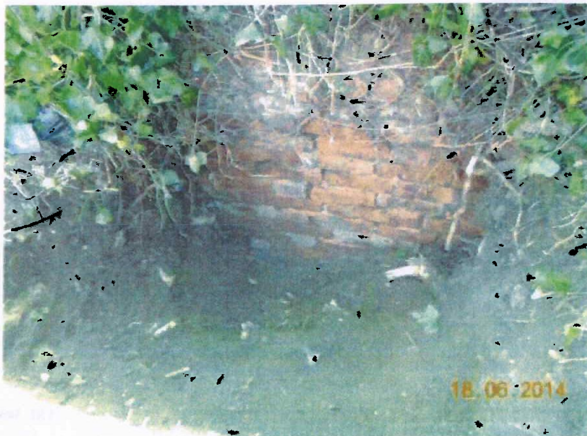
Photo No. 04 – Trial hole excavated behind wall
