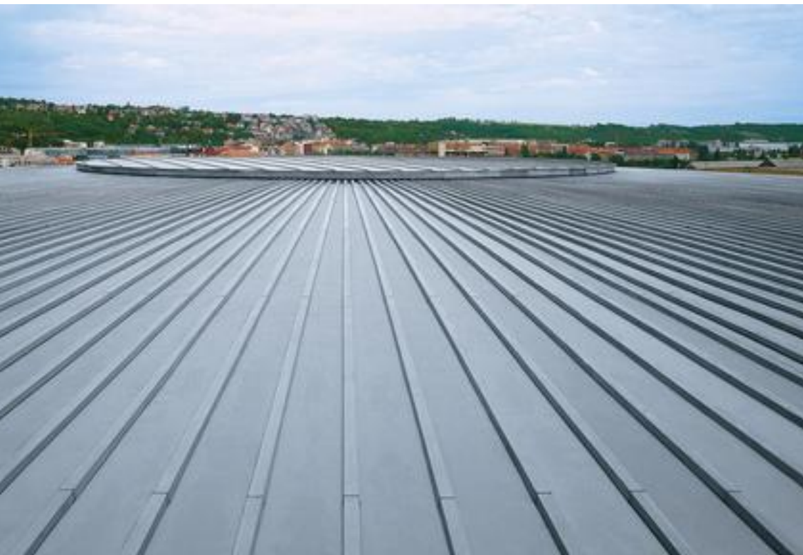
Example of Rheinzink zinc roof
