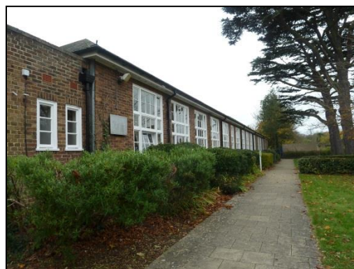
Figure 2 Facing south-east showing hardstanding pathway close to western boundary of site with introduced shrub
