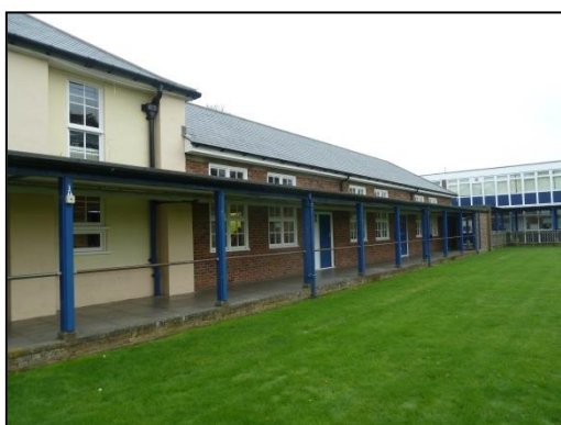
Figure 3 Facing north-west showing amenity grassland courtyard and surrounding buildings
