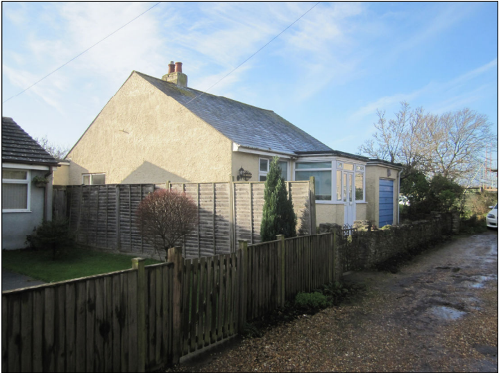
7. View of vehicle access and neighbouring property to East of site.
