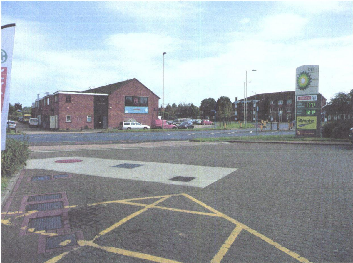
External views of the site: View towards to Purbrook Way;
