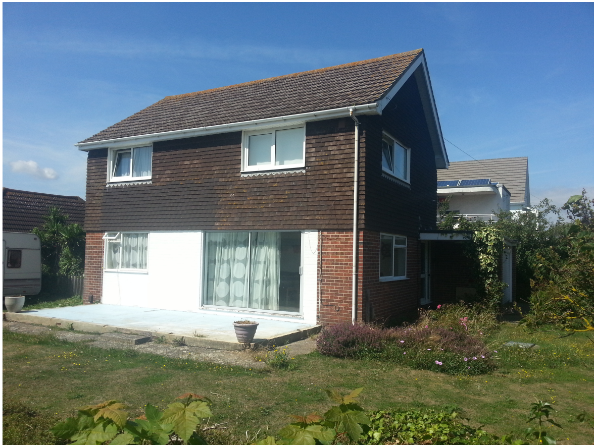
Fig 1: Existing side of House where part of the single storey extensions will sit.
