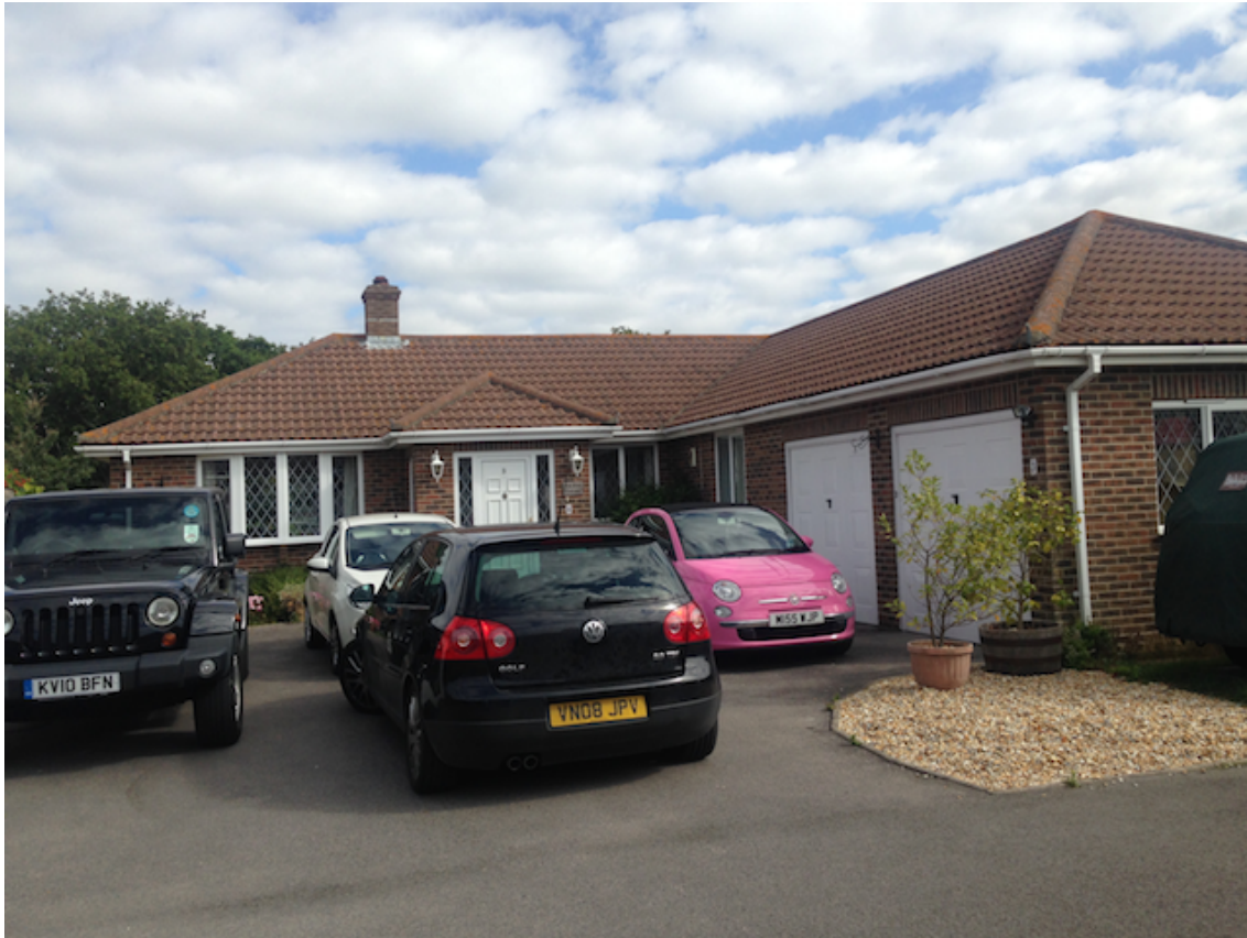
Figure 3. Front elevation of 3 Swans Walk showing the driveway and ornamental planting.
