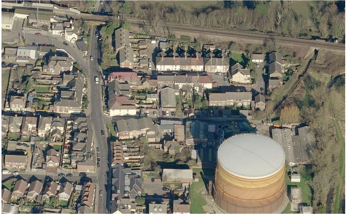
Aerial view of the Application site looking North
