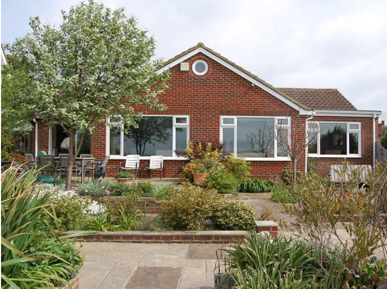
Figure 6: Rear elevation of the property
