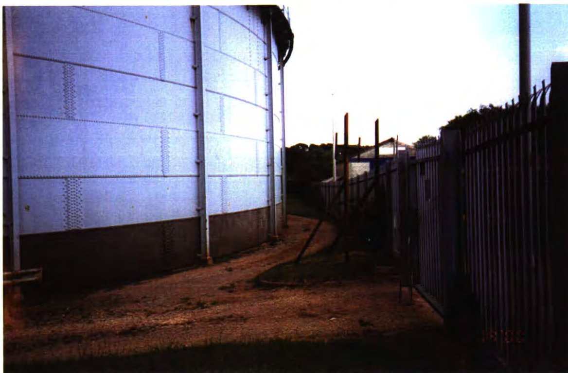
Photograph 2: Transco site area looking east along southern boundary, with doublegates at site entrance.
