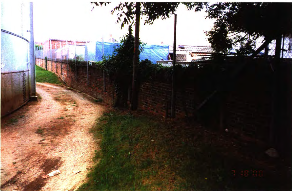
Photograph 8: Transco area looking east along northern boundary.
