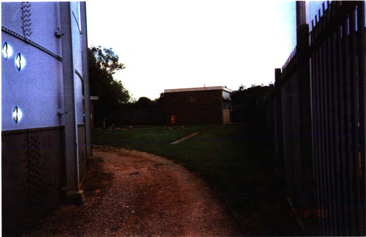
Photograph 3: Transco area looking east.
