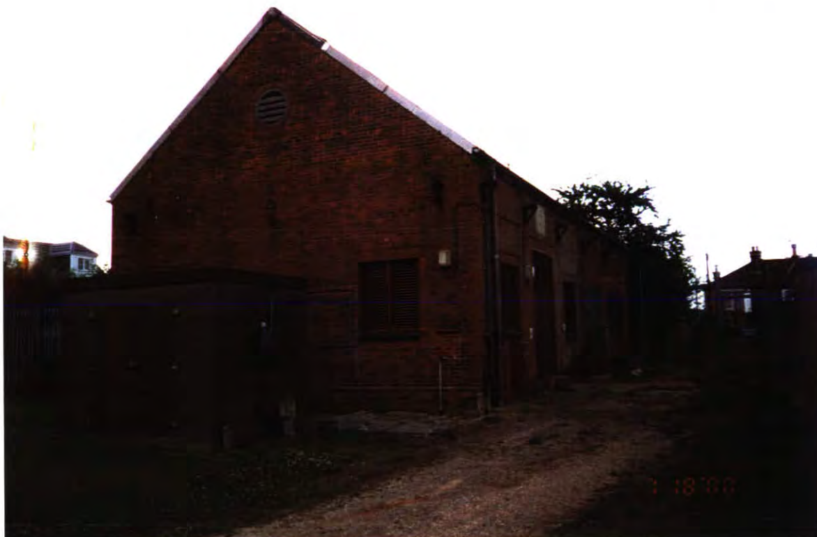
Photograph 5: Transco area – booster house.
