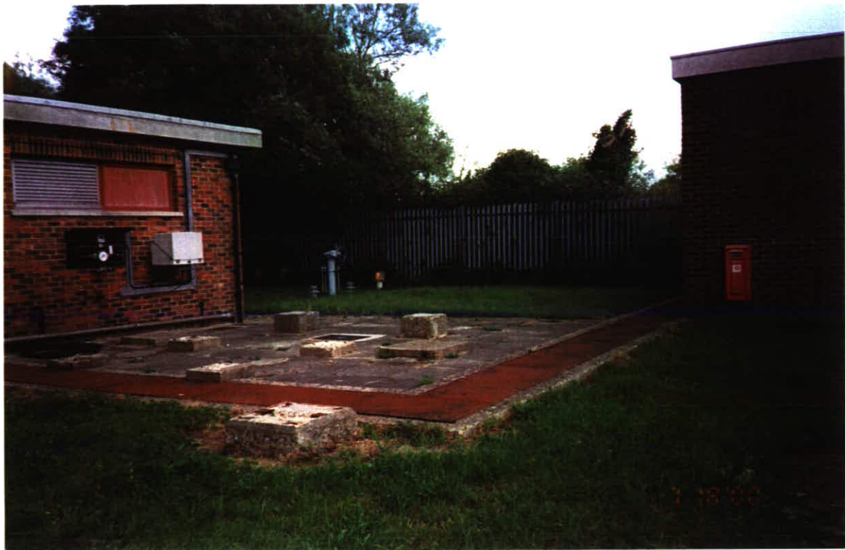
Photograph 11: Transco area looking northeast at the former structure base.
