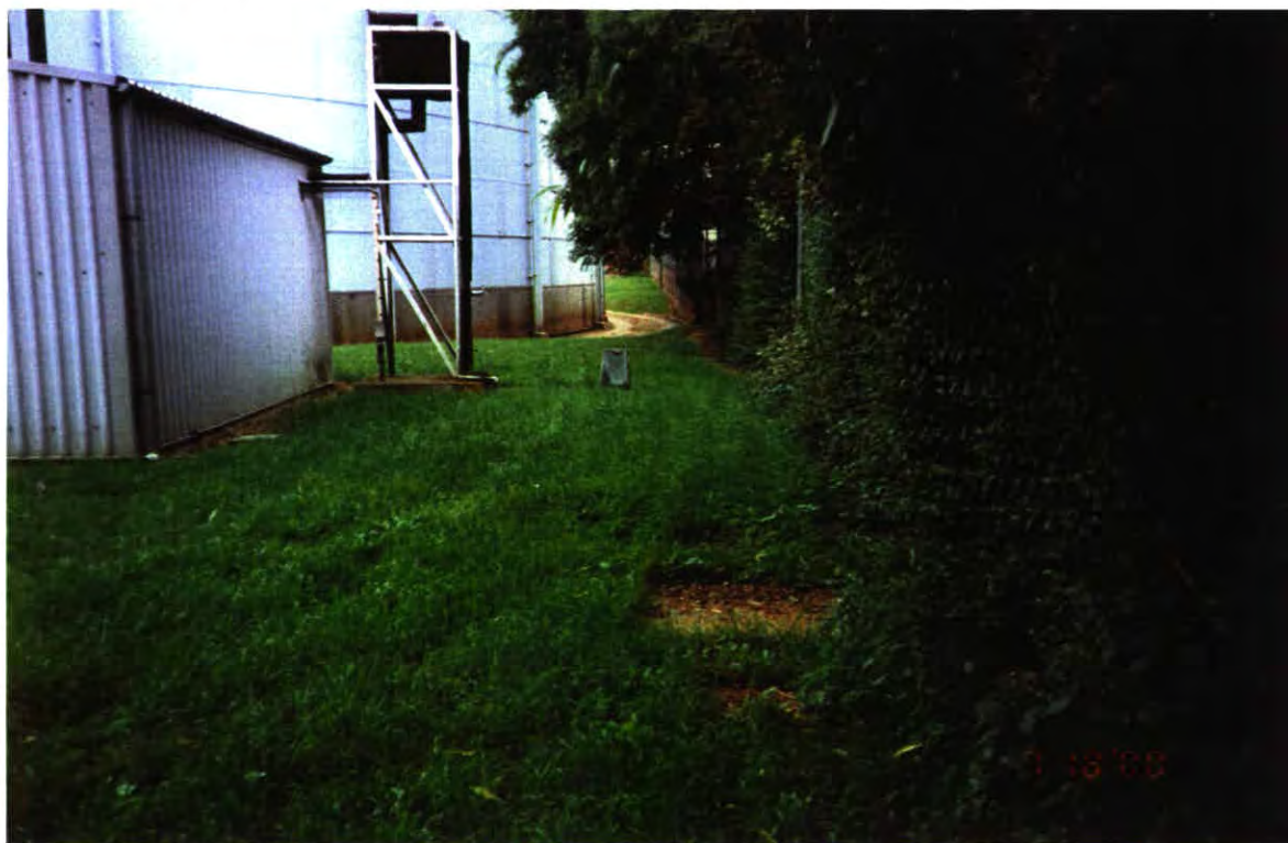
Photograph 6: Looking towards the gasholder from the northeastern corner of the site.
