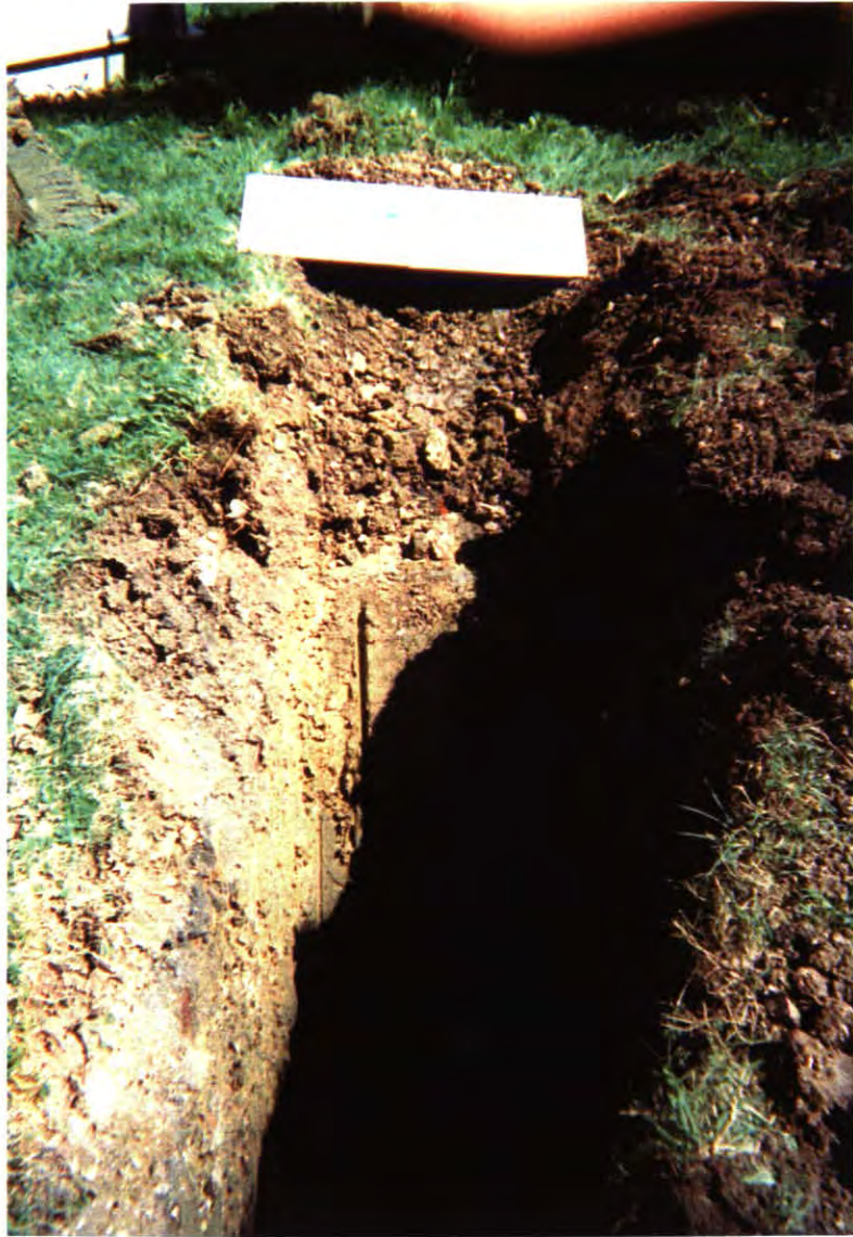
Transco SI Photograph 3: Showing trial pit TCTP4 eastern edge of pit, fill material inside former gas holder no. TC1
