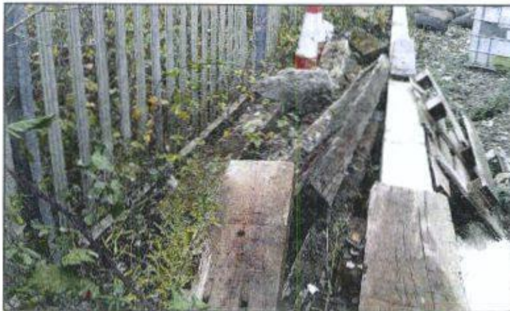
Photograph 2: Log sleeper pile in BG/TR1
