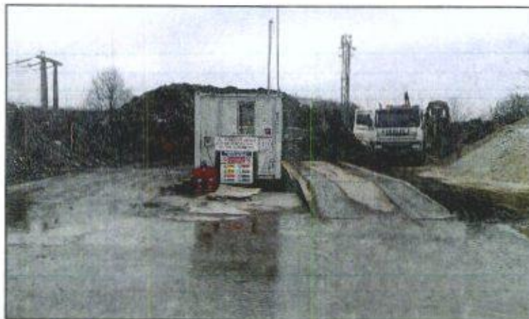
Photograph 3: Site weigh station (B3) and aggregate mound
