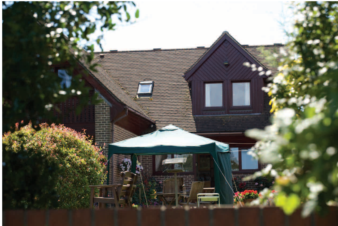
Photograph 13. 11D Salterns lane from 'My Lords Pond'. Type: Two Storey Property. Second storey within roof
