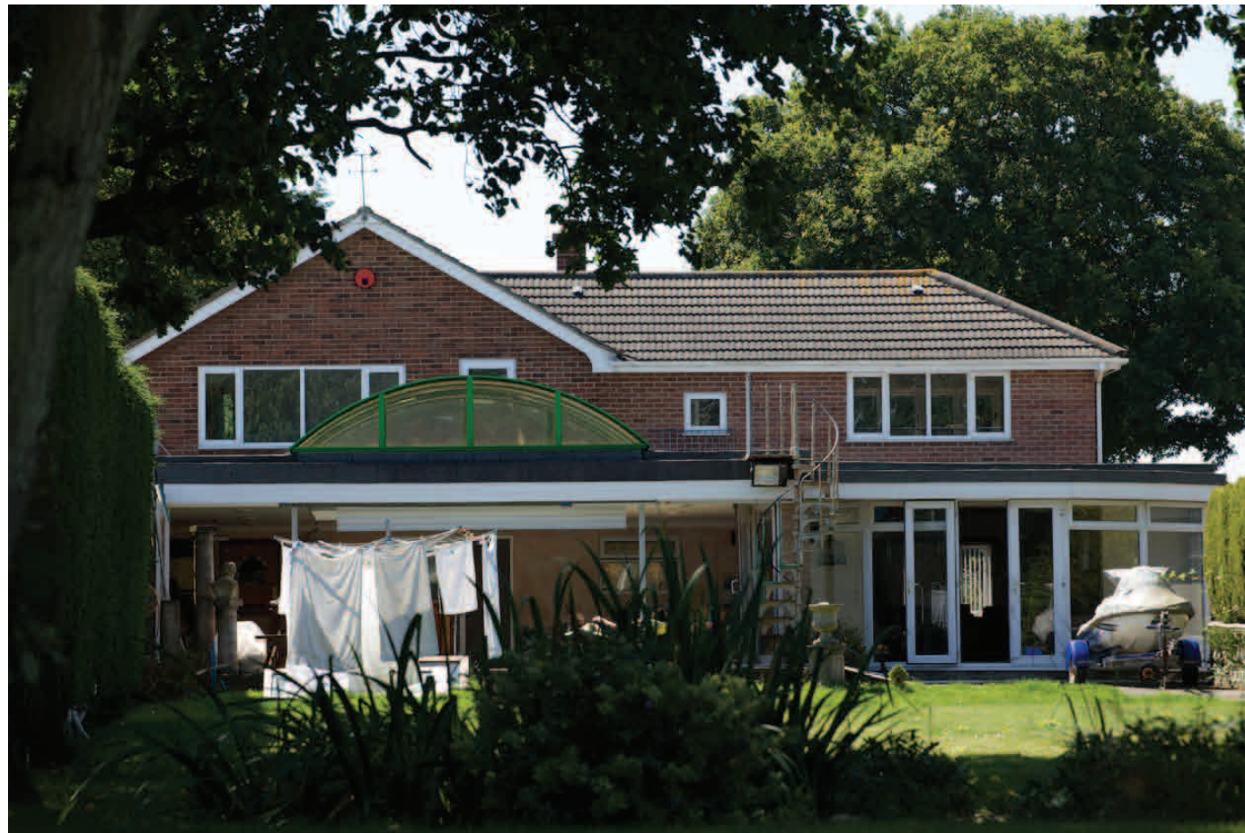
Photograph 1. 7 Salterns Close from 'My Lords Pond'. Type: Two Storey Property with pitched roof
