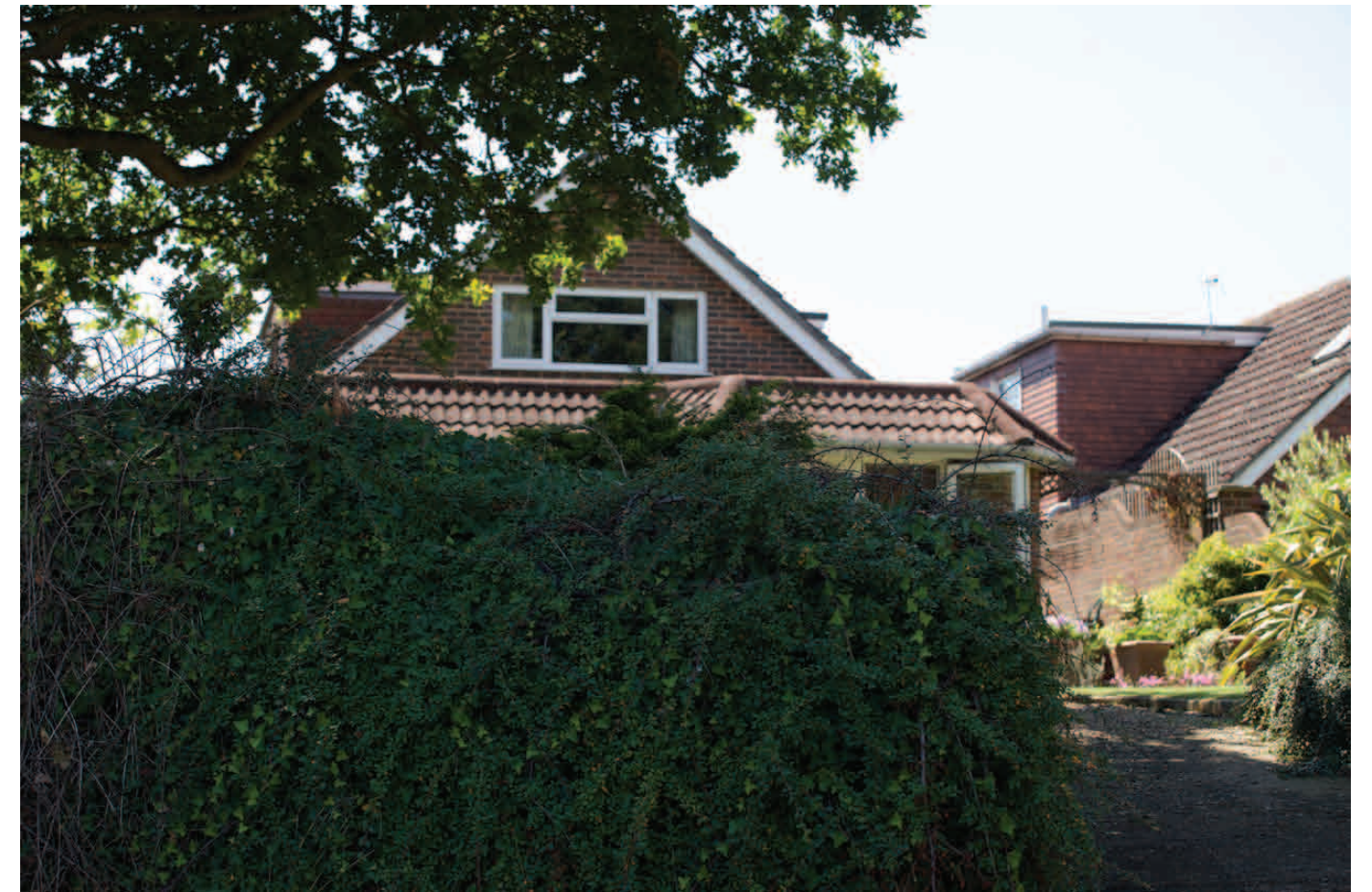
Photograph 19. 5a Simmons Green from 'My Lords Pond' Type: Two Storey Property. Second storey within roof
