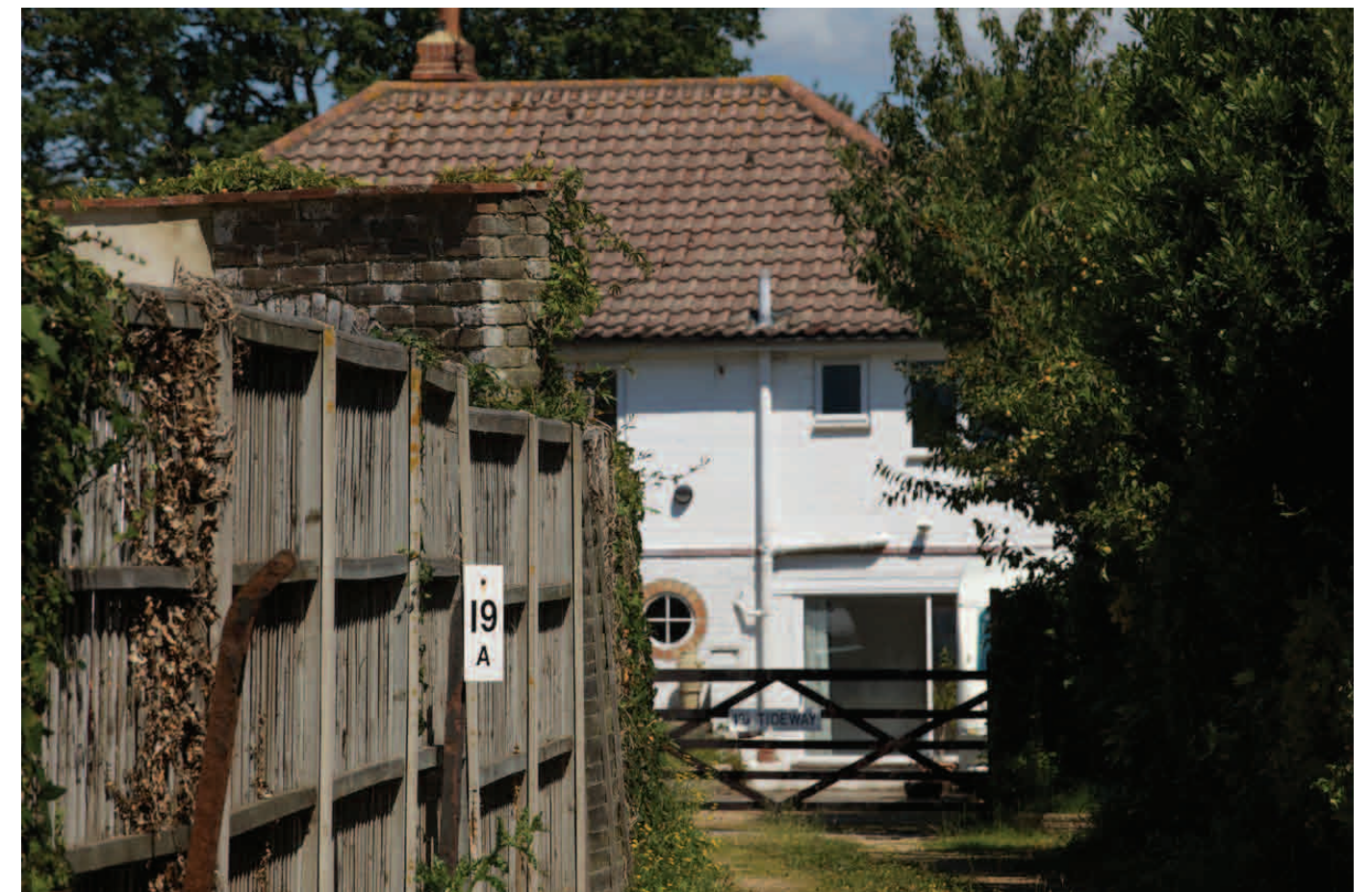
Photograph 12. 19a Salterns Lane from the road Type: Two Storey Property with pitched roof
