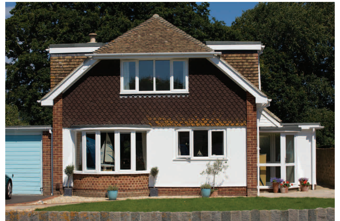
Photograph 8. 4 Salterns Close from the road Type: Two storey property. Second storey within roof/ dormer
