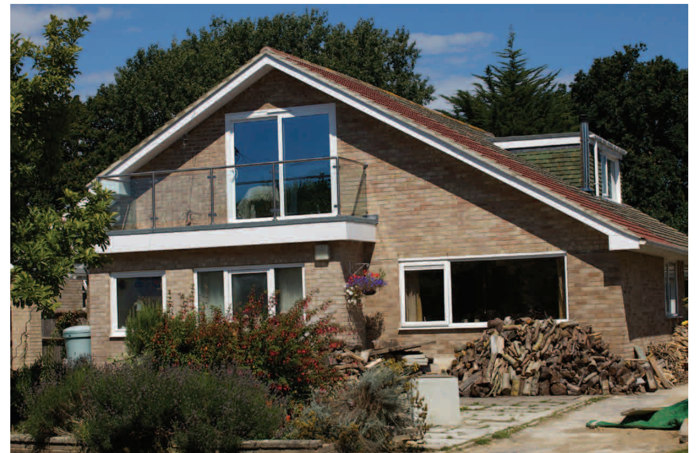
Photograph 4. 6 Salterns Close from the road Type: Two storey chalet property with pitched roof
