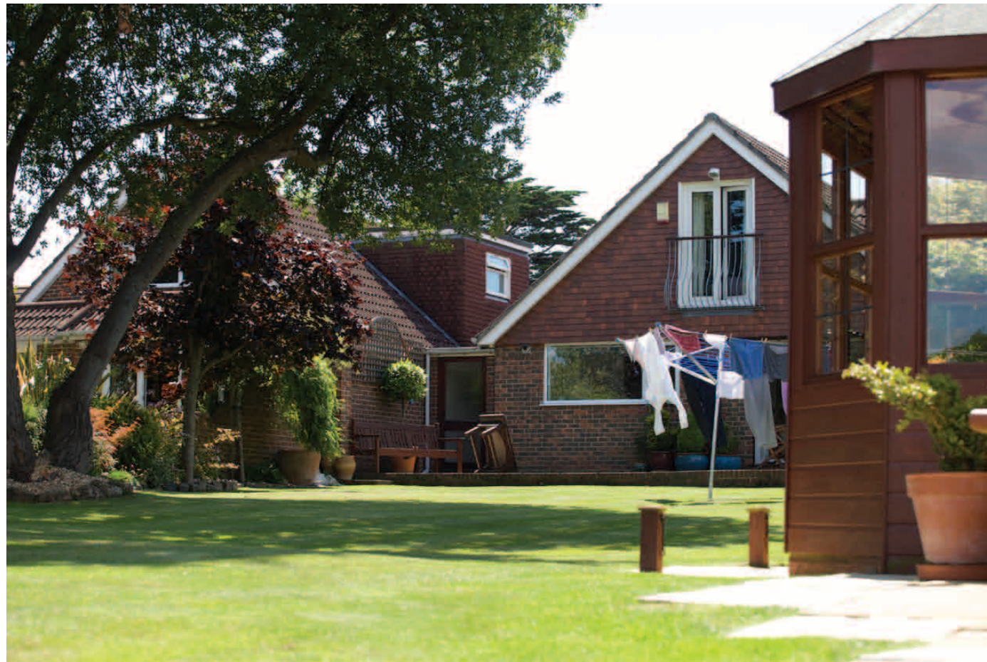
Photograph 21. 5&5a Simmons Green. Type: Two Storey Properties. Second storey within roof
