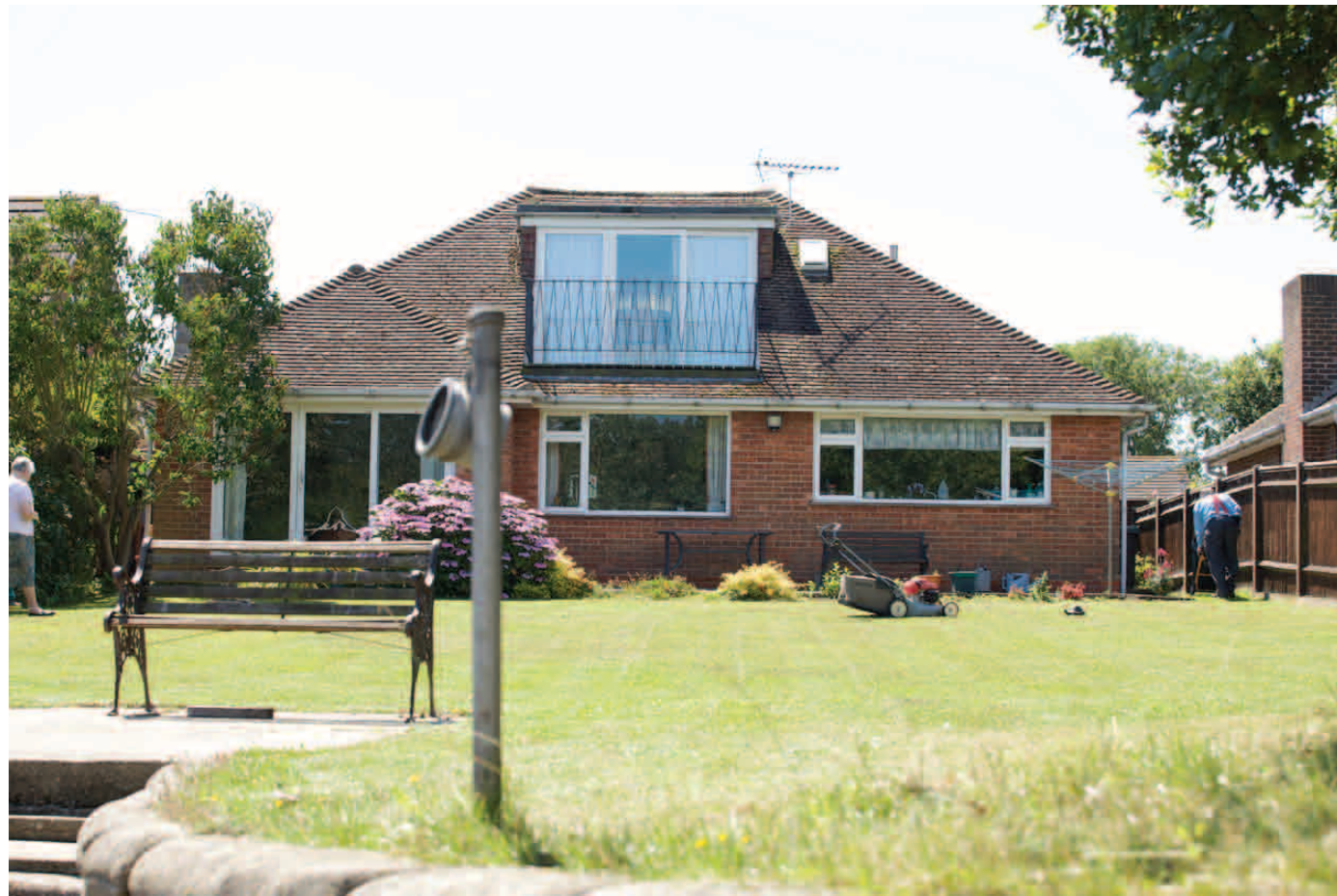
Photograph 25. 3 Simmons Green. Type: Two Storey Property. Second storey within roof
