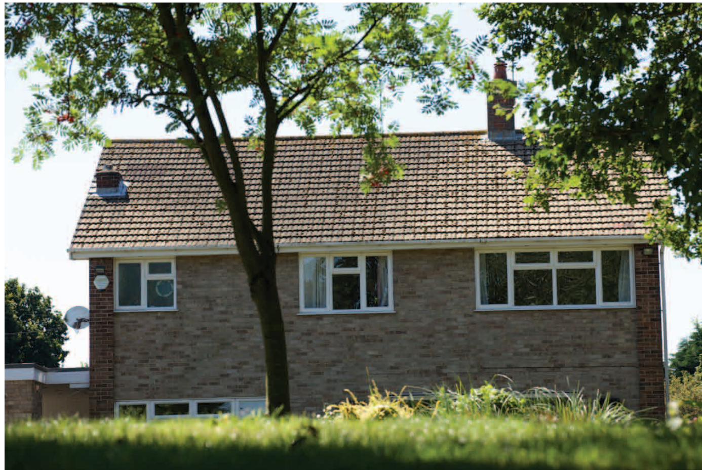
Photograph 5. 5 Salterns Close from 'My Lords Pond'. Type: Two Storey Property with pitched roof
