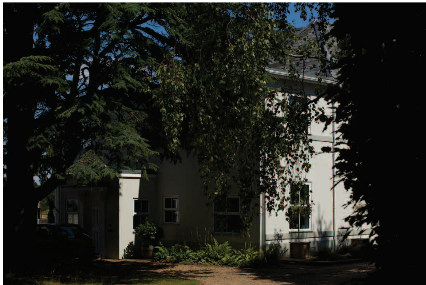
Photograph 10. Salterns House from the road. Type: Two Storey Property with pitched roof
