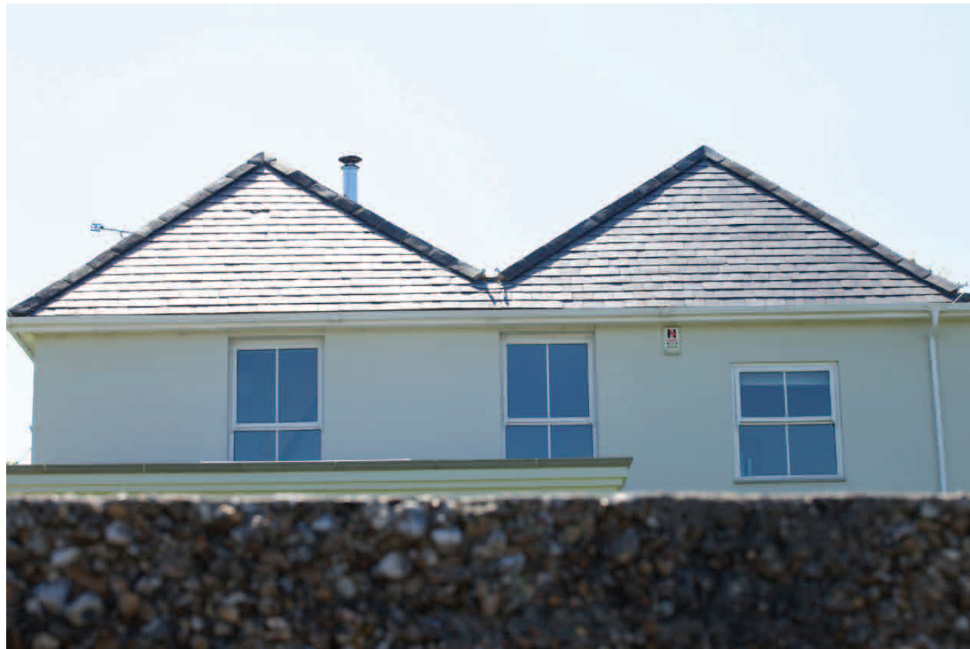
Photograph 9. Salterns House from 'My Lords Pond'. Type: Two Storey Property with pitched roof
