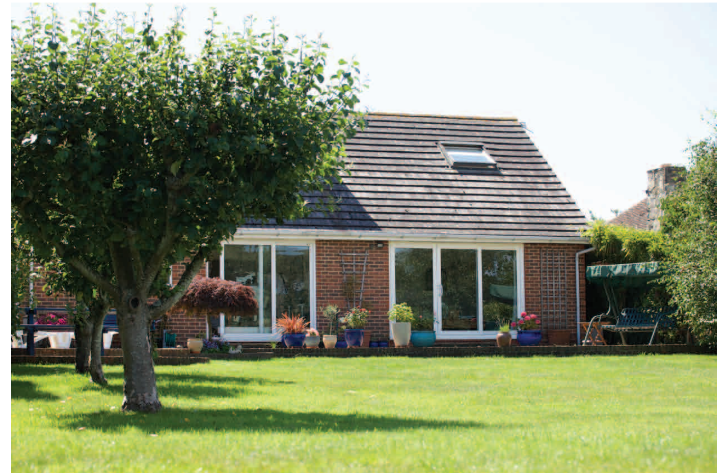
Photograph 23. 4 Simmons Green from 'My Lords Pond' Type: Two Storey Property. Second storey within roof
