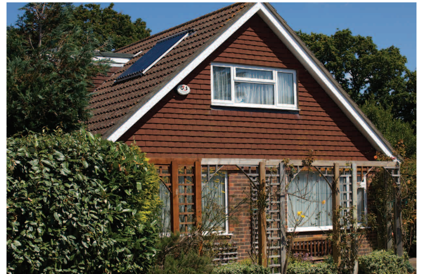
Photograph 20. 5a Simmons Green from the road Type: Two Storey Property. Second storey within roof
