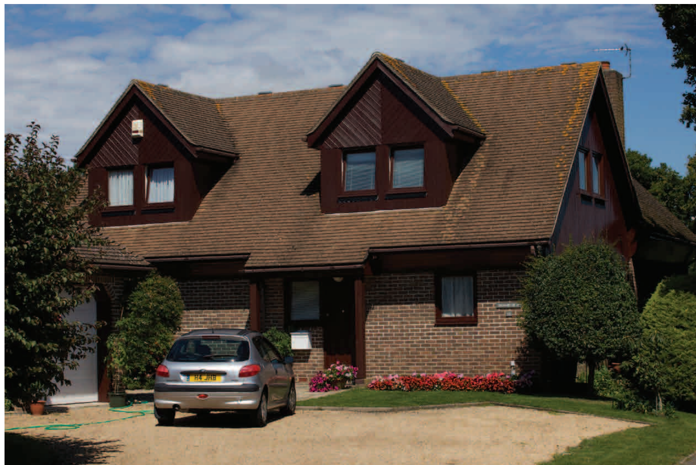
Photograph 14. 11D Salterns lane from the road. Type: Two Storey Property. Second storey within roof
