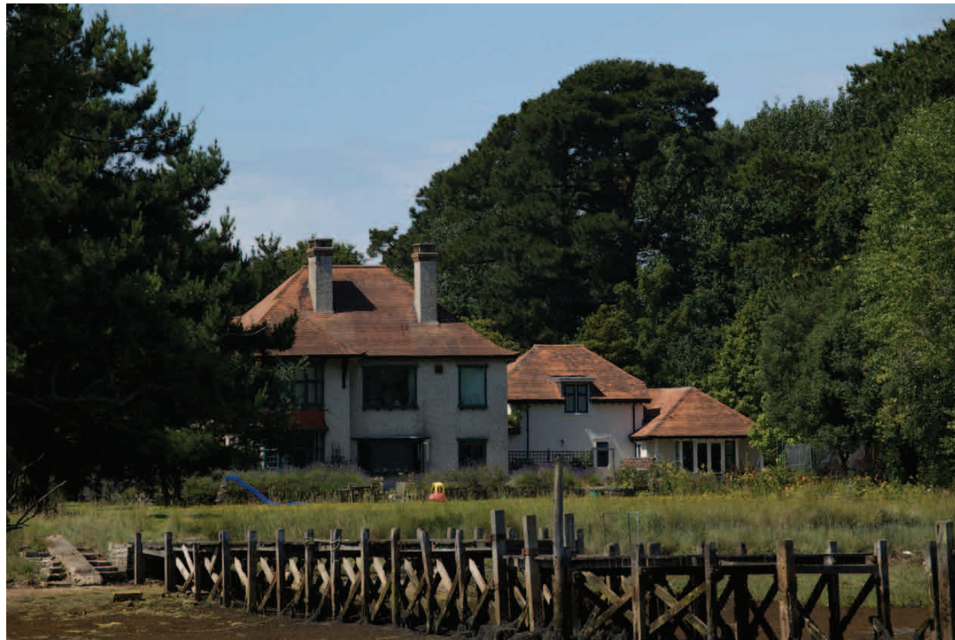
Photograph 30. Property to Western end of 'My Lords Pond'. Type: Two Storey Property.
