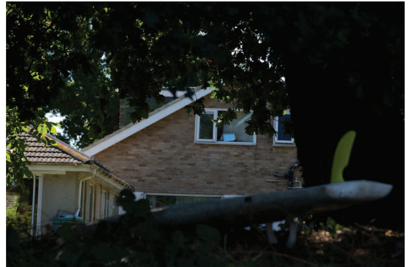
Photograph 3. 6 Salterns Close from 'My Lords Pond' Type: Two storey chalet property with pitched roof
