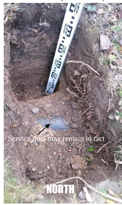
Trial Pit 2 (South East)
