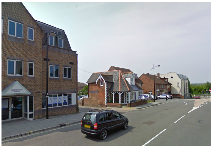
Site looking North towards no. 9 & 11 St. Georges Walk, with the turning for Portland Road just visible.
