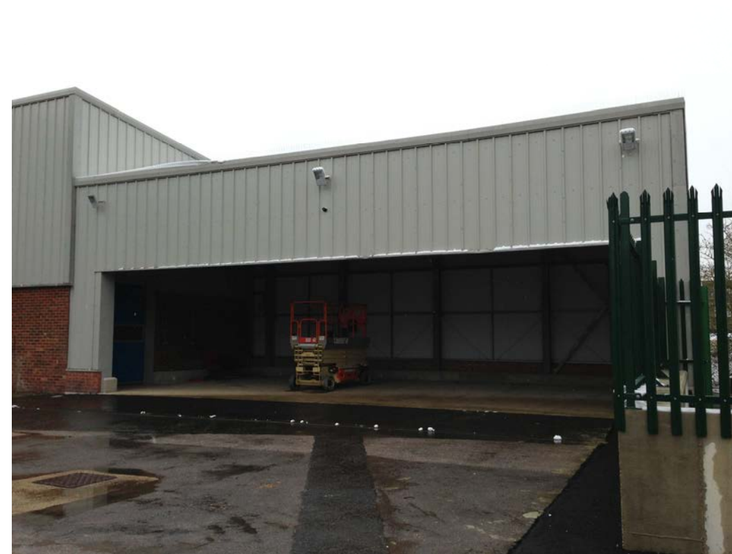
Existing building part of loading bay
