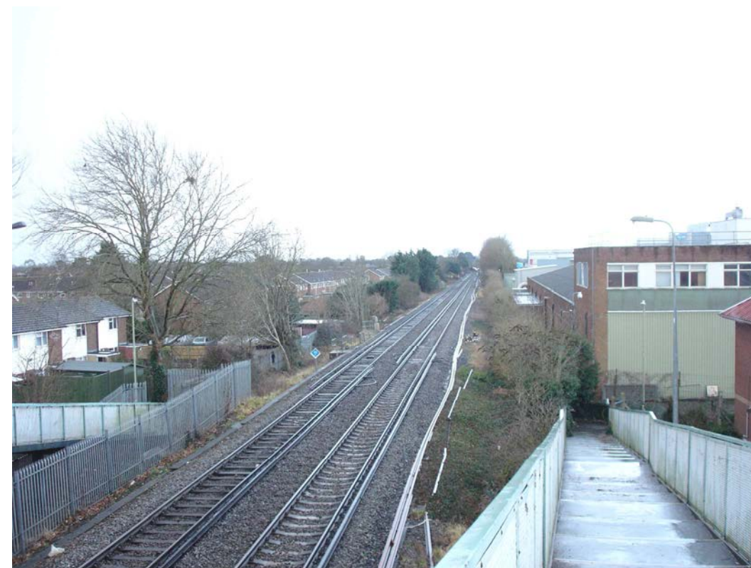
Site and surroundings viewed from the footbridge
