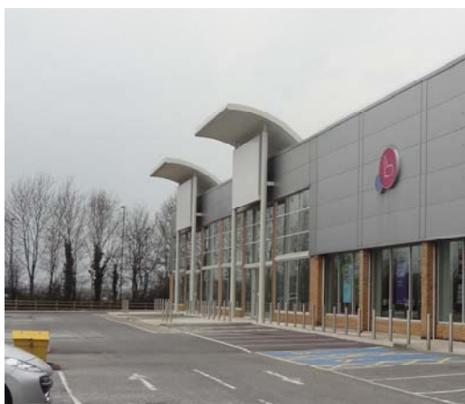
Recently completed extension to DFS block showing palette of materials and entrance canopy
