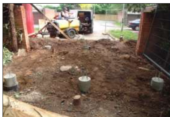
Photo 41: Piles can also be used to support bridges across sensitive RPAs, but the temporary ground protection has to be removed before the main structure is either imported in or cast on site.
