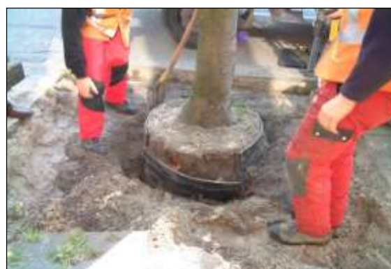
Photo 58: This excavated tree shows the root deflectors that were installed when it was planted seven years previously. The product has deflected roots downwards and prevented damage to the adjacent surfacing. Note that this is a permeable sandy soil and the roots were able to grow beneath the bottom of the deflectors.
