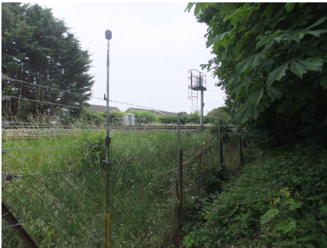
Photo 4 Long term monitor at the railway site boundary
