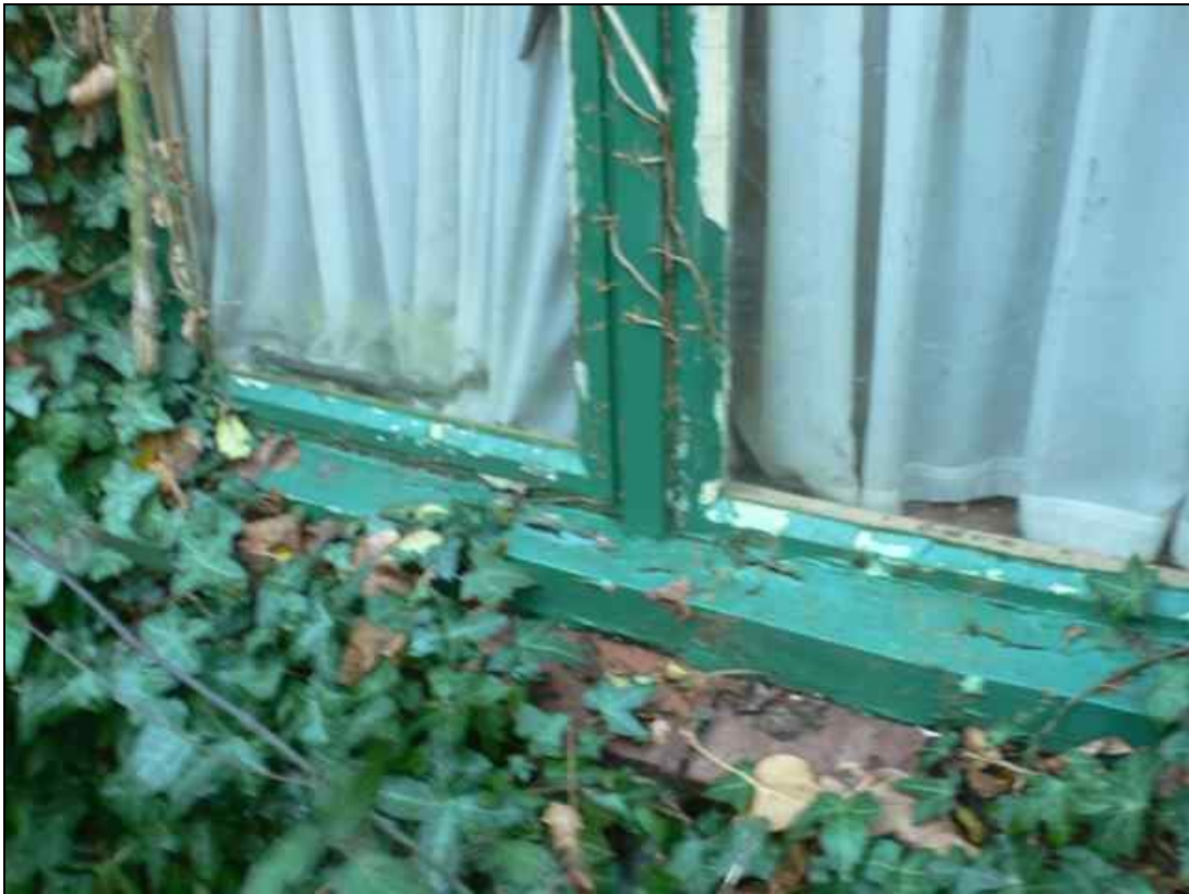
Photo 12 All external surfaces of the structure were assessed for evidence of bats such as bat droppings. No evidence of use was noted.
