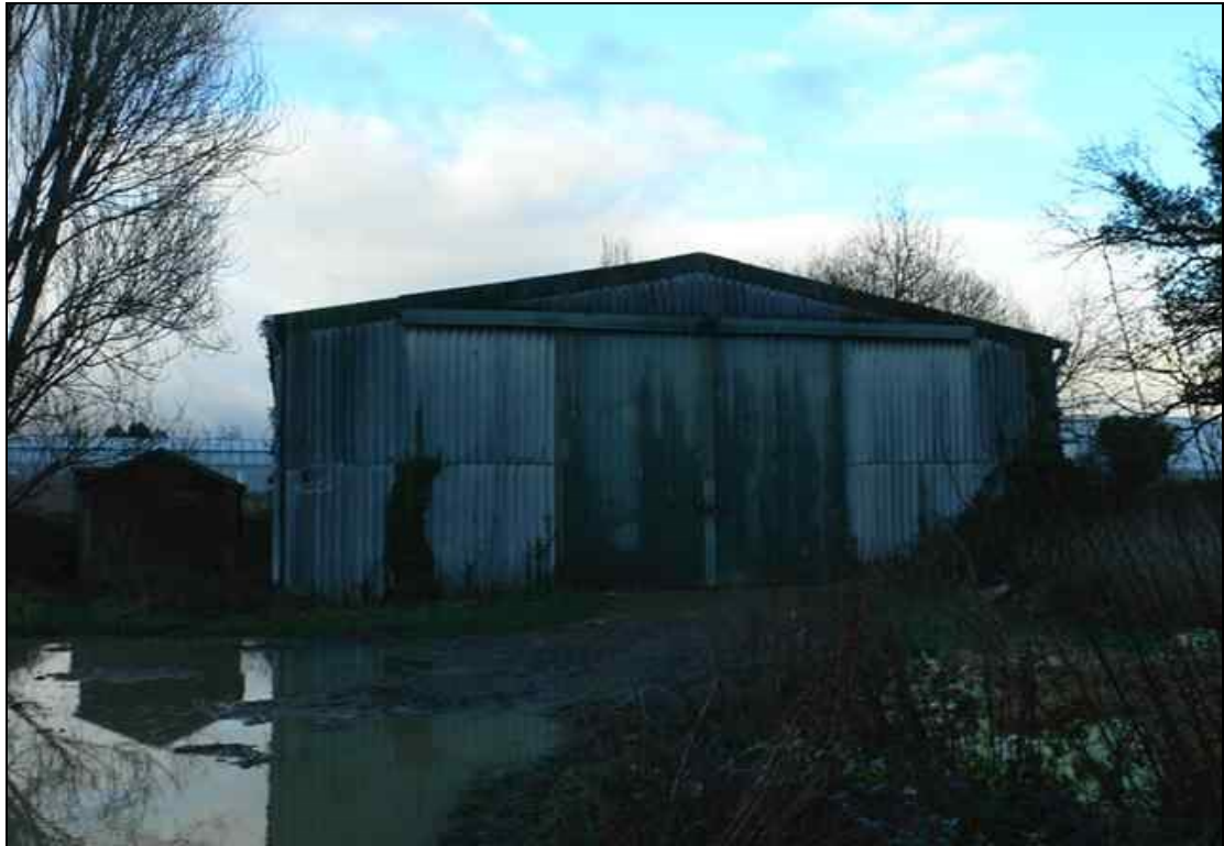
Photo 18 The outbuildings are predominantly of corrugated iron construction on a timber frame with limited roosting opportunity.
