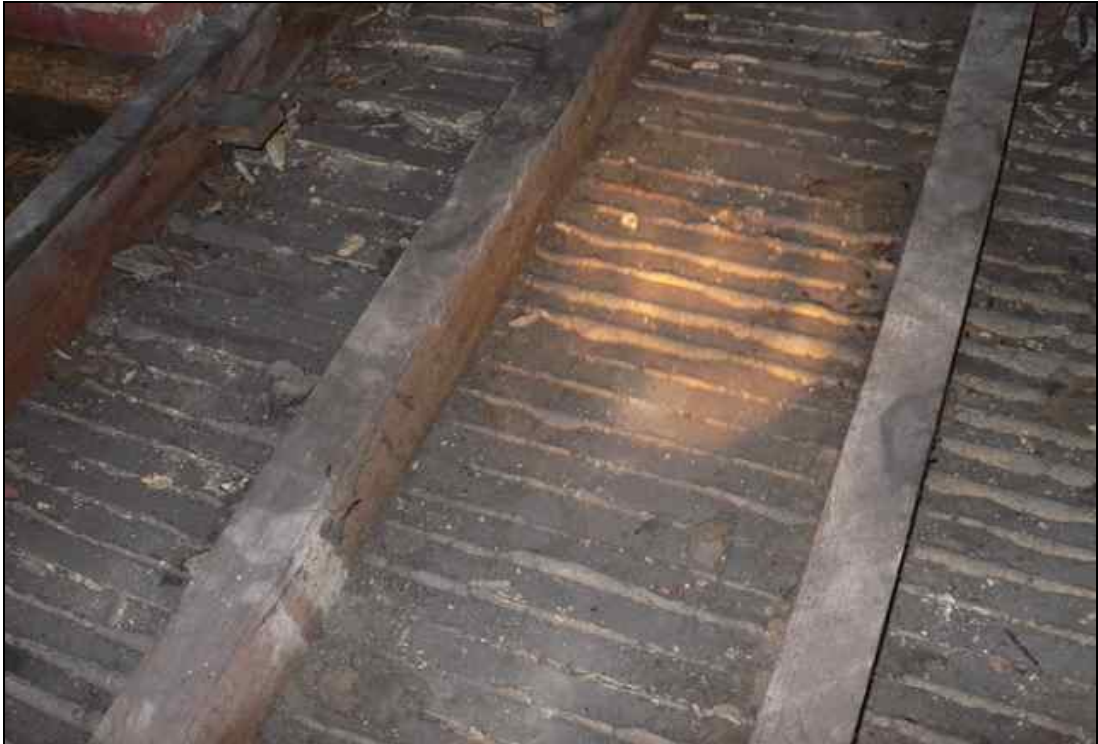
Photo 16 All surfaces of the structure were examined for evidence of bats such as bat droppings.
