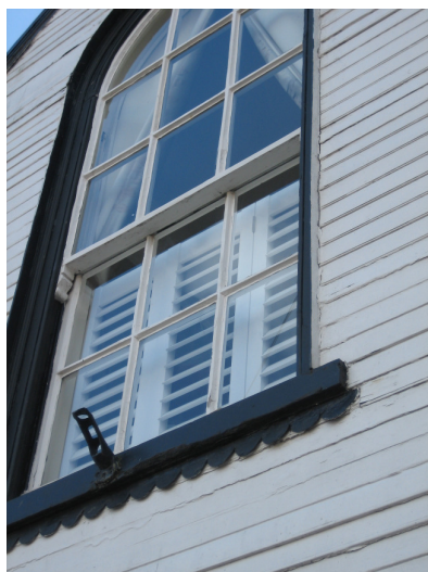
Fig 2 – View of window W5 – centre arch
