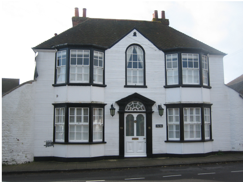
Fig 1 – Principal northern facade of The Hut along King Street...
