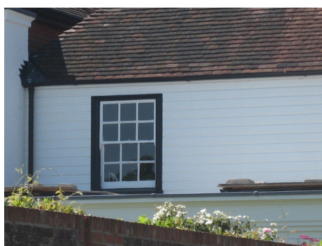
Fig 4 – First floor side window to East elevation
