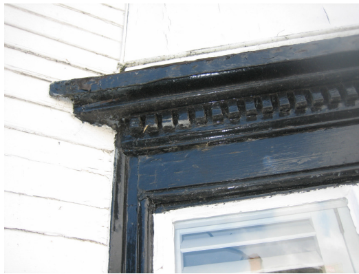
Fig 5 – View of the existing cornice/dentil course above bay windows
