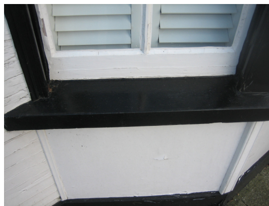
Fig 3 – View of existing bay window W1a - cill
