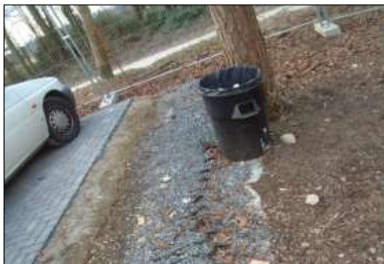
Photo 26: A conventional concrete haunching can be used to retain new surfacing as long as it is not dug into a trench - here is it placed on top of the CellWeb layer.
