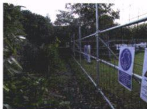
Example of protective fencing:
